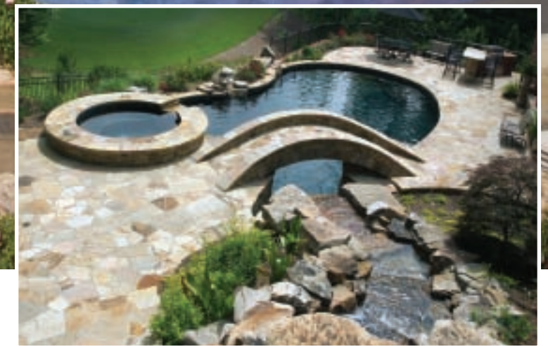
A little bit of heaven. By taking advantage of a severely sloping yard, an upper streambed was designed so that water could flow over different elevations, under the bridge and into the pool. The dark pebble finish used on the pool's interior offers a reflective quality.
